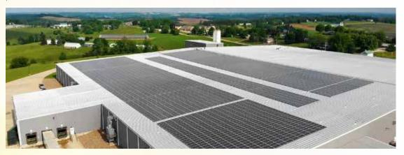
In 2021, we completed installation of a 1.792 MW solar array at our stone manufacturing facility, comprised of 4,480 solar panels. It is expected to reduce electrical power consumption by 60% and to prevent emission of 1,472 tons of CO2 annually.
